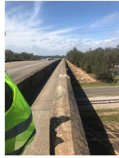
Very narrow ped/bike lane over bridge
